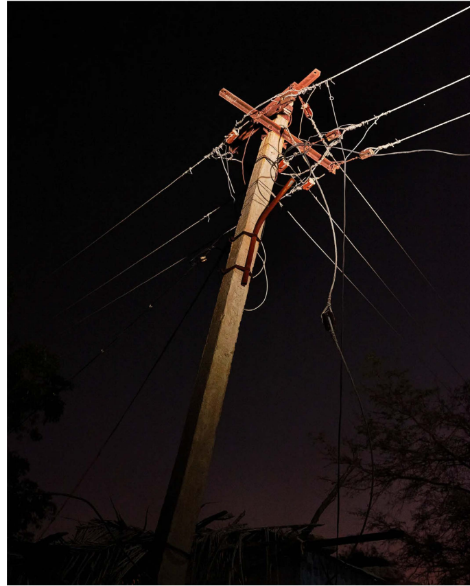
A newly constructed electrical pole in Vollur village, near Pavagada Ultra Mega Solar Park.
