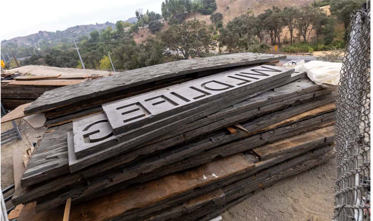
Concrete molds for new signage on the Wallis Annenberg Wildlife Crossing. (Brian van der Brug / Los Angeles Times)
