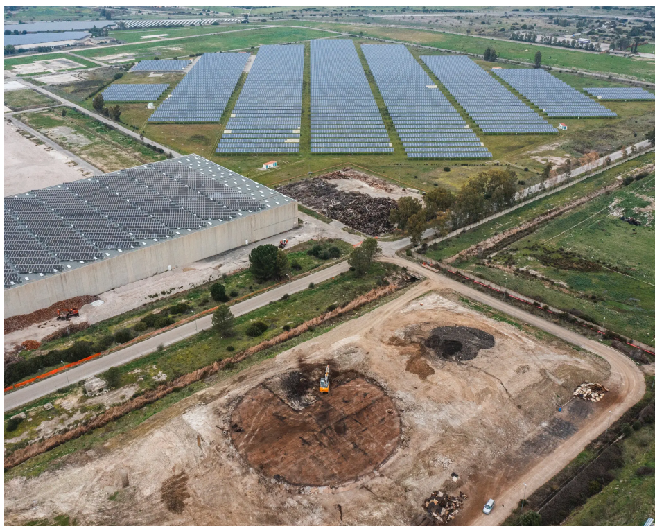
The site in Ottana of the future full-scale version of Energy Dome's battery. Gaia Squarci for The New York Times
